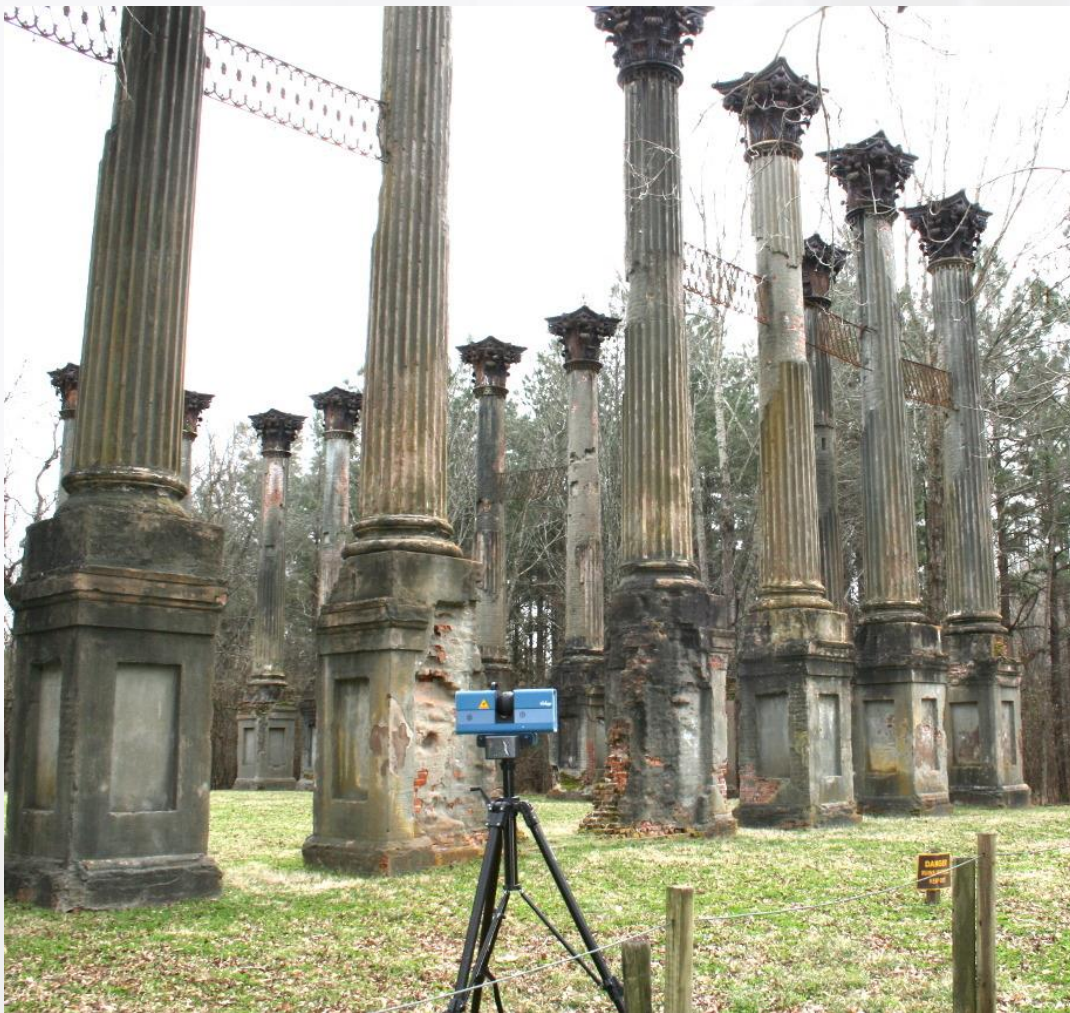
3D Scanning all 23 columns to generate a high resolution rendering and 3D model
